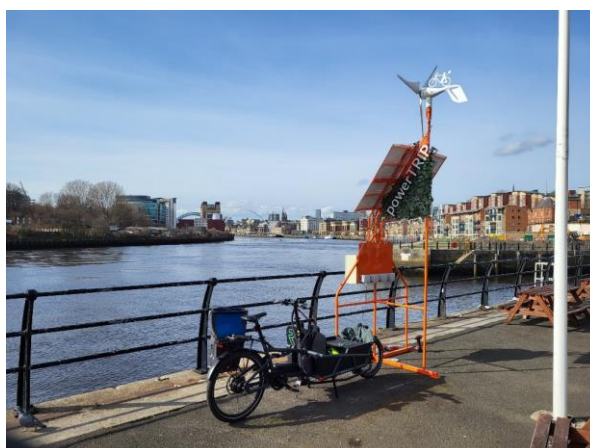
E-bike charging point on Newcastle's Quayside
